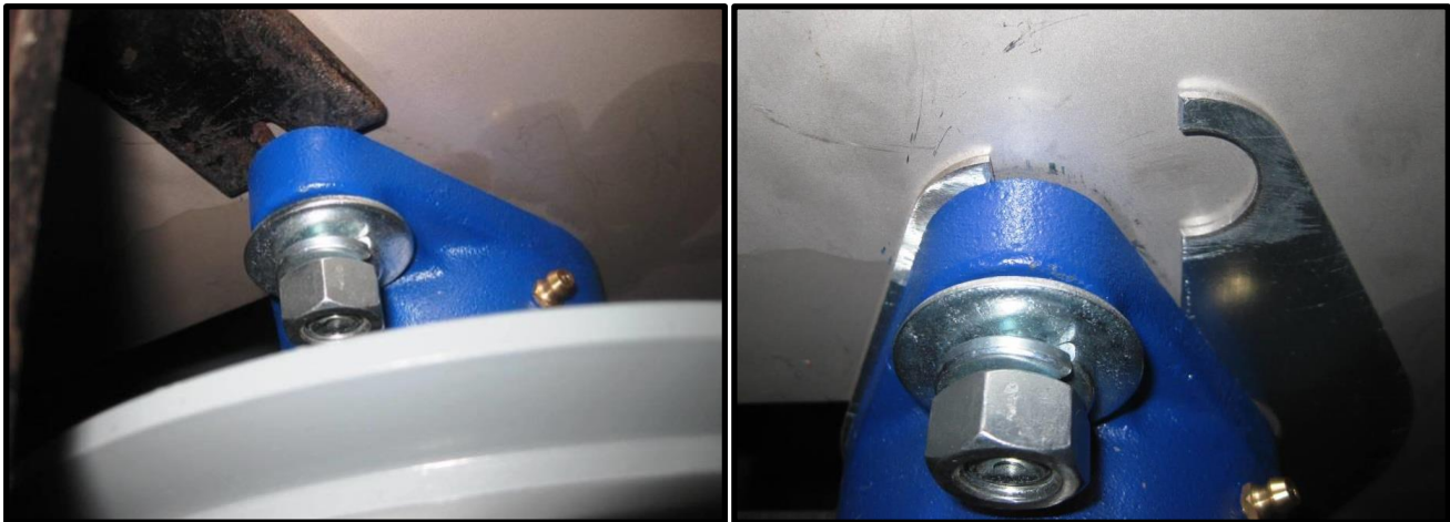
Figure 6- Installing shim plates
